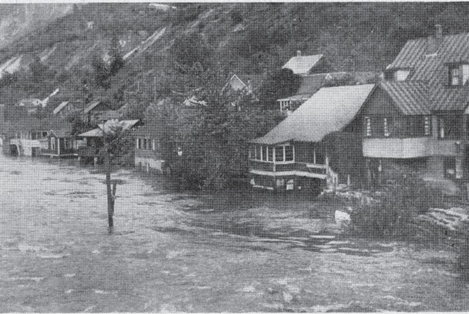
Here are the houses on Bay avenue on the Trail side of the bridge across the Columbia river. Downstream from the bridge they are under to the height of the bottom story. Great damage has been done but the worst is believed over. (Photo by Dale Morgan, staff photographer of The Spokesman-Review.)
