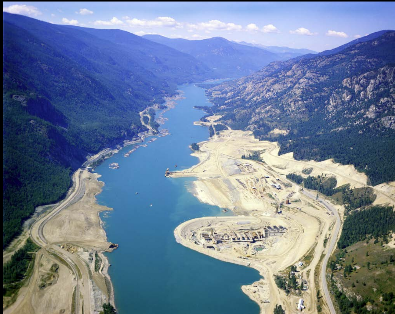
High Arrow Dam (renamed Hugh Keenleyside Dam)
